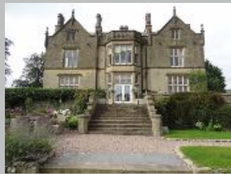
S elevation of Falcon Manor Hotel
