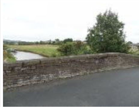
View north Eastwards from Horse Close Bridge over canal
